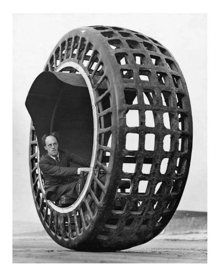
In 1930 John Archibald Purves created a gyrocar called the Dynasphere. It consisted of a 450kg iron latticework built like a wheel with a small petrol-powered engine. The device was steered by the driver leaning in the desired direction of travel...
