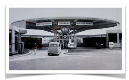
and featured a cantilevered canopy. Now here's the thing. In 1963 the garage proprietor installed Britain's first selfservice petrol pumps. Three of the pumps were designed to blend five intermediate grades of petrol, the remaining six delivered the two standard grades available at the time. With no pump
